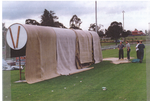
Source: Murray Neish Figure 3. 1220 mm duct - wrapped with carpet
