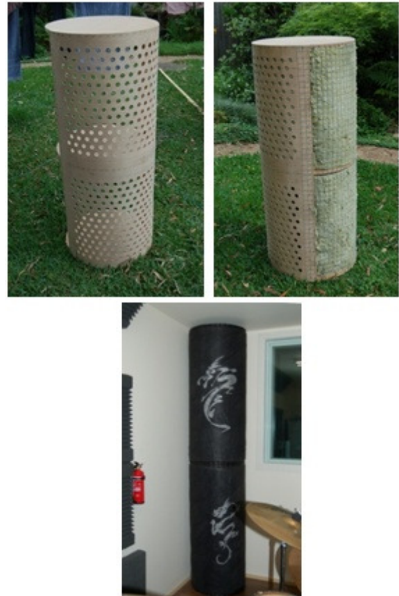
Figure 11 Construction Details of Tube Traps; Plywood Frame (upper left); With Rockwool Infill (upper right); Corner Installation in Studio (bottom)
