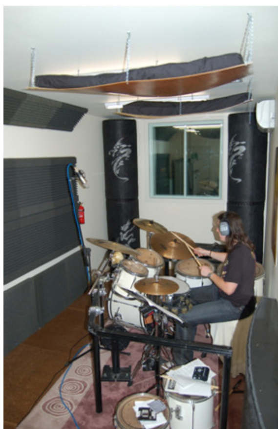
Figure 18 Photograph of Drum Studio Interior Demonstrating Key Absorption Treatments
