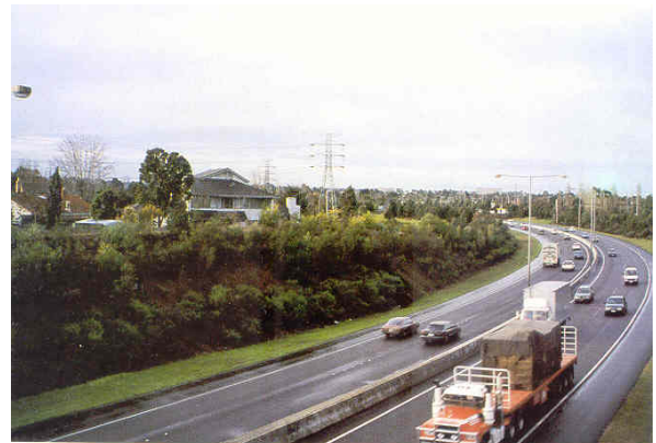
Figure 4. Embankment and Freeway Source: (Hong Kong EPA 2003)
