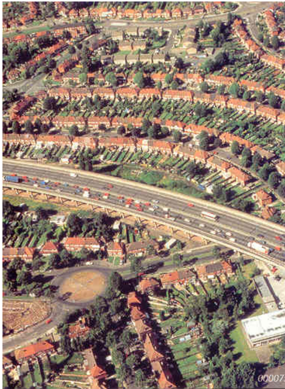
Figure 8. Residential development having acceptable façade sound insulation
