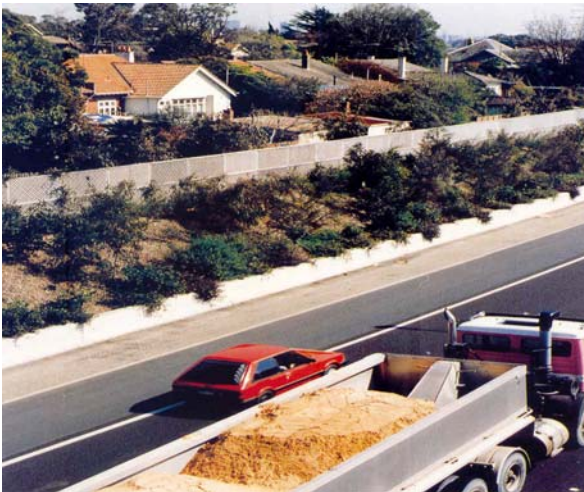
Figure 7. Noise barrier system providing acceptable acoustical performance Source: (Roberts 2003)
