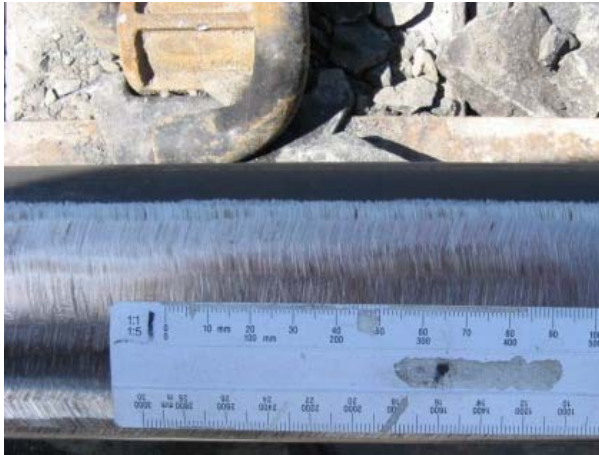
Figure 7: Scratch marks visible on rail head immediately after grinding
