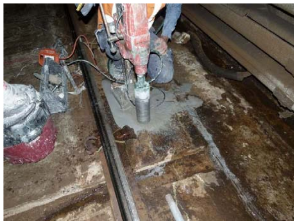
Figure 5: Core drilling an existing track slab to investigate remaining design life
