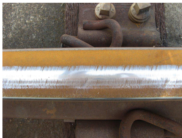
Figure 6 Photo of the rail head near the noise test site, showing the clear running band
