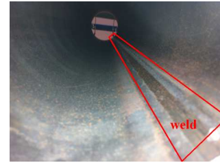
Figure C1: The welding line in the cylinder
