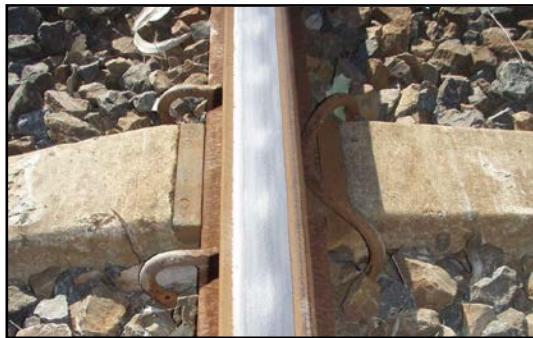
Figure 1 - 9-month-old corrugated rail profile
