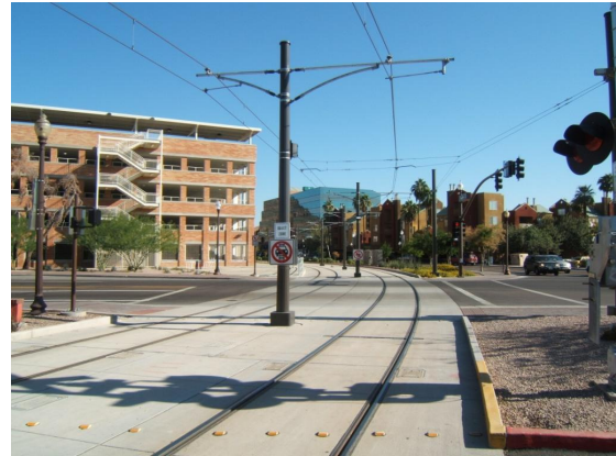
Figure 8. Curve near Hayden Square Condominiums
