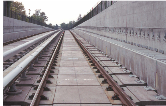
Figure 2. Floating Slab Trackbed at BART
