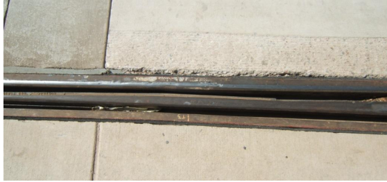
Figure 5. Example of Rough Running Rail (at top)
