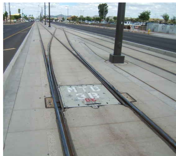
Figure 4. Single Crossover of Embedded Track
