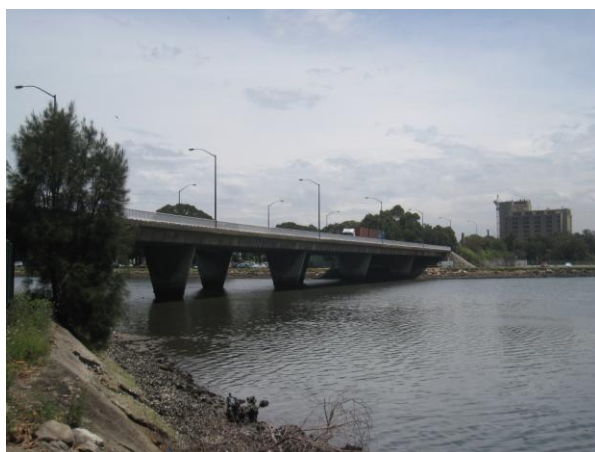
Figure 13. Bridge B, showing the size of the pylons.
