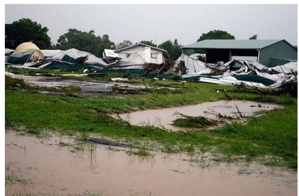
Figure 3. Flood damage (Source: The Courier-Mail)
