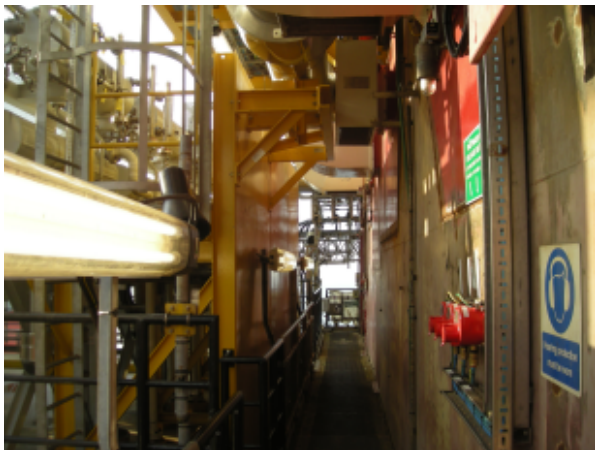
Figure 11: Steel wall screening access walkway from fan coolers.
