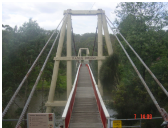
Figure 4 - View of Kane's Bridge, Kew Victoria
