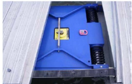
**Figure 13** Tuned Mass Damper
