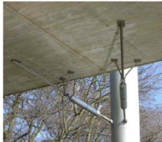
**Figure 12** Viscous Damper
