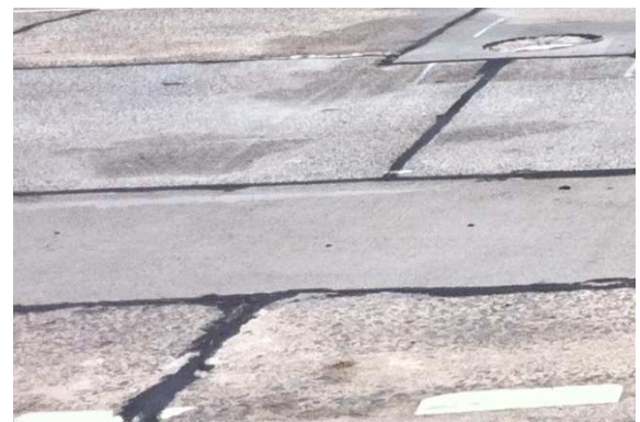
Figure 18. Road 4 – Post DG
