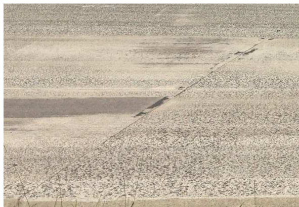
Figure 13. Road 3 – Post DG works
