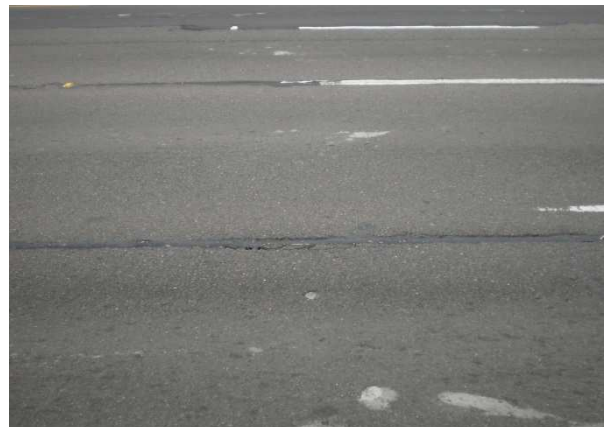
Figure 1. Road 1 – Pre rehabilitation works
