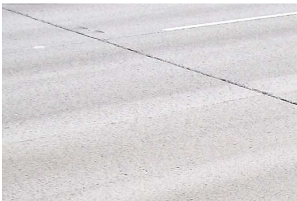
Figure 7. Road 2 – Post DG works
