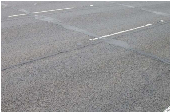
Figure 6. Road 2 – Pre rehabilitation works
