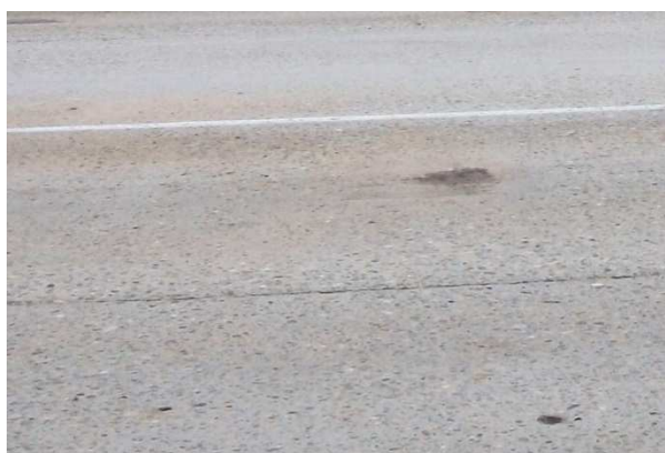
Figure 3. Road 1 – Post SM works
