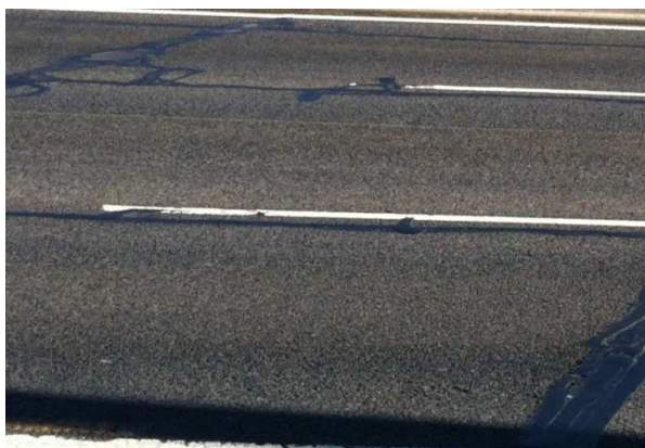
Figure 11. Road 3 – Pre rehabilitation works
