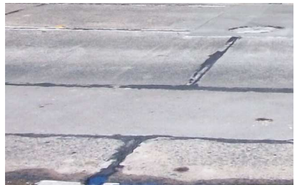
Figure 17. Road 4 – Pre Works
