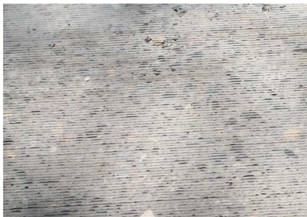
Figure 2. Road 1 – Post DG works
