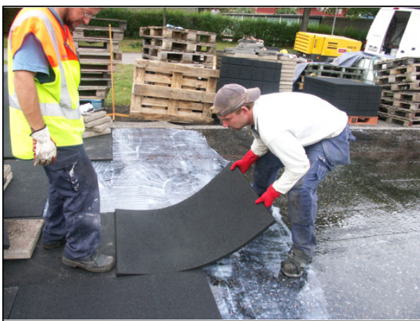
Figure 1. Mounting of rubber panels in 2004 on a street in Stockholm.
