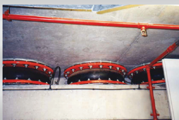
Swimming Pool Air Spring Supports
