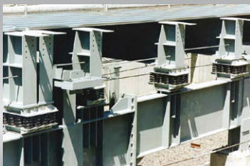
Spring Isolators Close to Railroad
