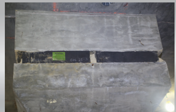
Low Dynamic Stiffness Building Isolation Bearings at Column Capital
