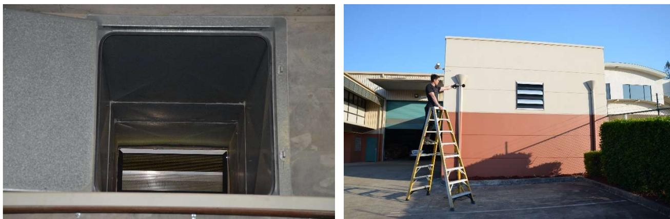
Figure 7: Metal duct and flush mounted louvre flush with the wall at end of duct
