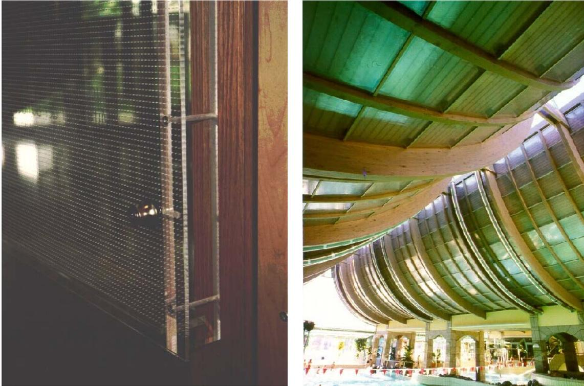
Figure 3: Application of micro-perforated panel absorber (MPA) as an acrylic glass panel (left) with overall thickness of 50 mm and polycarbonate foils on swimming pool at 130 mm, double layer set-up (right)..
