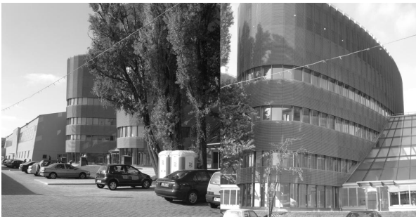
Figure 3. Complex of new buildings of Wyższa Szkoła Menedżerska in Warsaw after completion – on the left: recreation centre; in the middle: two office buildings, classrooms, two small lecture halls; on the right: building with the main auditorium, senate room, and two small lecture halls
