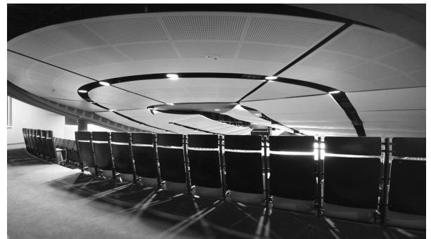
Figure 9. Spread fan-shaped perforated panels at the rear of the auditorium
