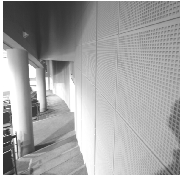
Figure 12. Arrangement of acoustic materials in side aisle area: view on semi-perforated Decogips modules covering concrete wall
