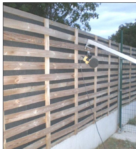
Figure 9. Barrier that doesn't meet minimum dimension requirements.
