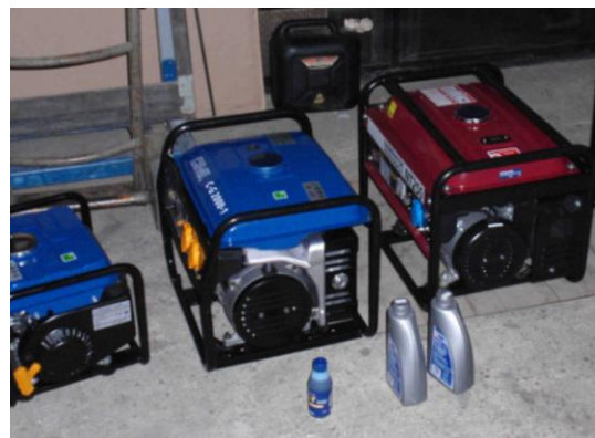
Figure 1. Gasoline engine-generators prepared for acoustic measurements
