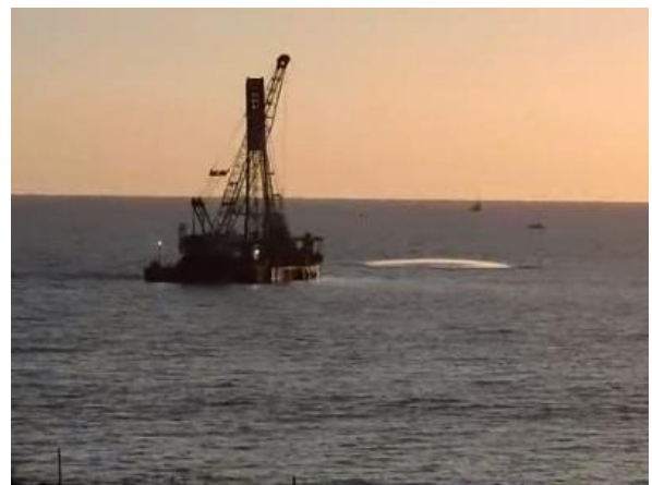
Figure 1. Blast effervescence near the shot-firer's barge off the coast at Binningup. The effervescence shown here was caused by a blast 12 times larger than the blast examined in the present paper.
