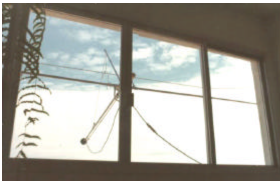
Photo 3. Window with an aluminum frame, two fixed and two sliding panes with a 3mm monolithic glass
