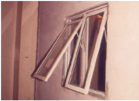
Photo 6. Window with an PVC frame and two projecting and sliding panes with a 3mm monolithic glass
