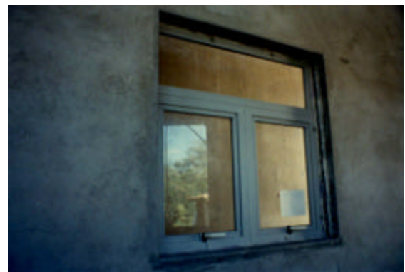
Photo 5. Window with a PVC frame, a fixed pane and two projecting and sliding panes with a 3mm monolithic glass. Sample assembled outside the laboratory (See Figure 1)
