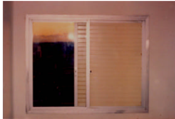
Photo 2. Window with an aluminum frame and three sliding parts, one with a 3mm monolithic glass and two blinds, made of plastic, for darkening and ventilation
