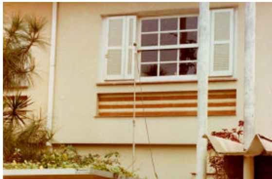
Photo 1. Window made of wood and 3mm monolithic glass
