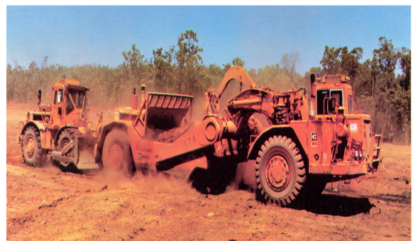
Figure 1. Bottom dump scraper stripping soil and gravel Source: (Alcoa 1982) [5]
