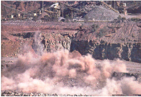
Figure 4. Construction blasting Source: (Cedric 1982)
