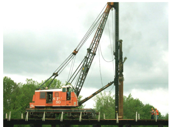
Figure 3. Impact pile driver
