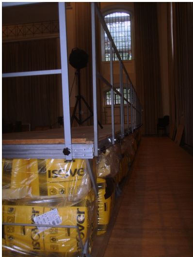
Figure 3. Dense porous material installed under the rostrum
