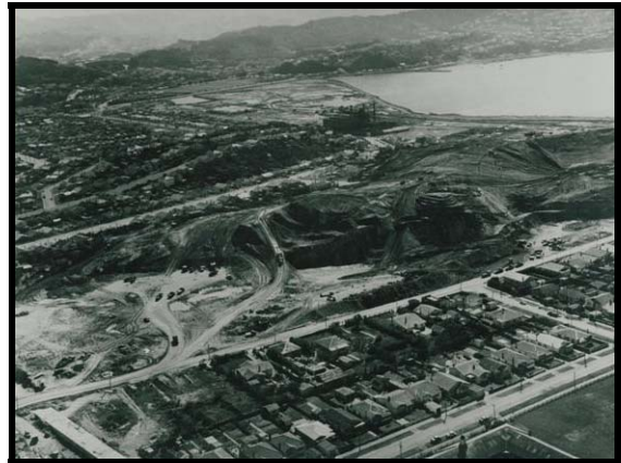
Figure 3 – Vast earthworks and the dissection of a suburb were required to develop Wellington Airport. The houses in the fore- and backgrounds still exist today.
