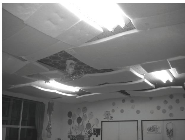
Figure 1. Installation of sound absorbing board
