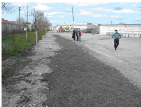
Figure 9. A vibroinsulation joint in the enterprise's territory between the source of vibration and the residential houses. It is 4.5 m deep and about 100 m long. A vibroinsulation joint is filled with keramzit granules.
