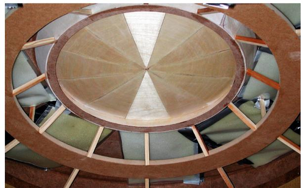
**Figure 18.** Membrane absorbers inserted in the roof of the auditorium.
