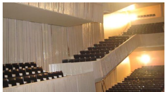
Figure 10. The horizontal diffusers installed in the 1:10 scale model hall
