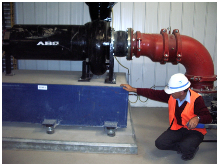
Figure 5. Photograph of installed cooling water pump, with inertia base on spring mounts and flexible connection to pipe work.
