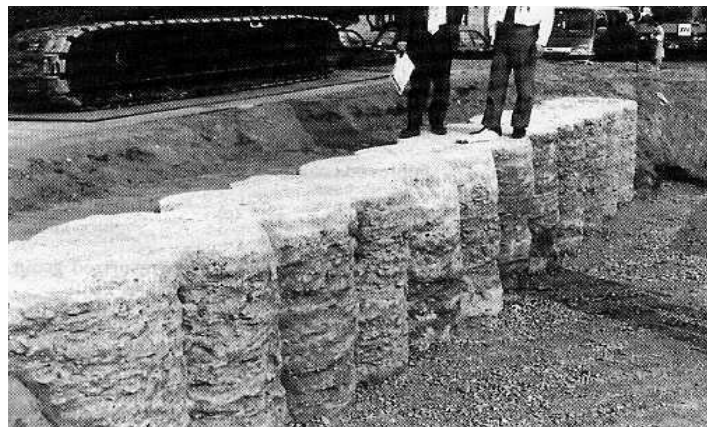
Figure 3. Deep mixing technology: treated ground in Japan
