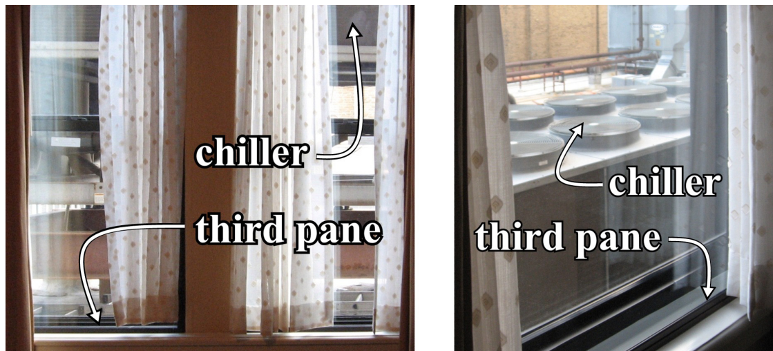
Figure 5. Interior views of triple-pane systems No.2 (left) and No.3 (right).
