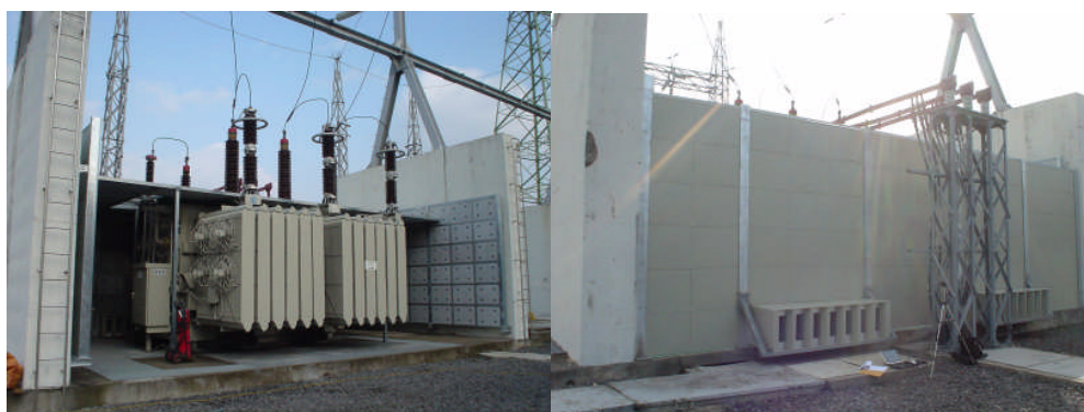
Figure 7. Installation of Partial enclosure
