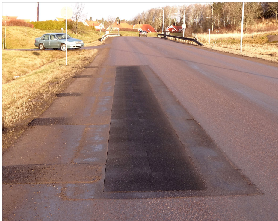
Figure 3. The 25 m long and 1 m wide test strip of PERS mounted on a local street in Linköping, Sweden. It covers the right wheel track of the traffic (which runs towards the viewer).
