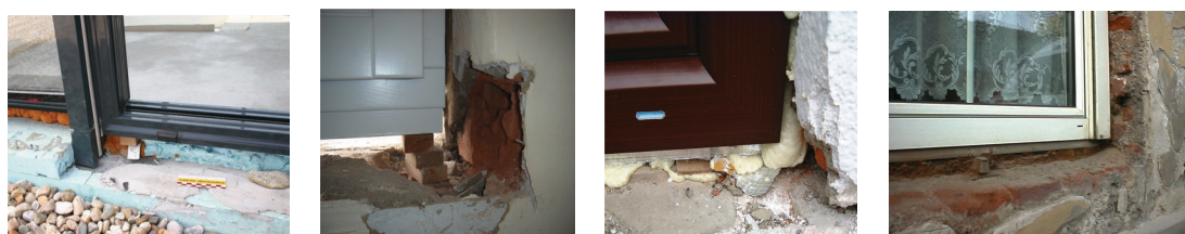
Figure 4 –building refurbishment: bad window mounting examples
