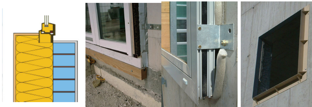
Figure 4 –window mounting in the insulation layer
