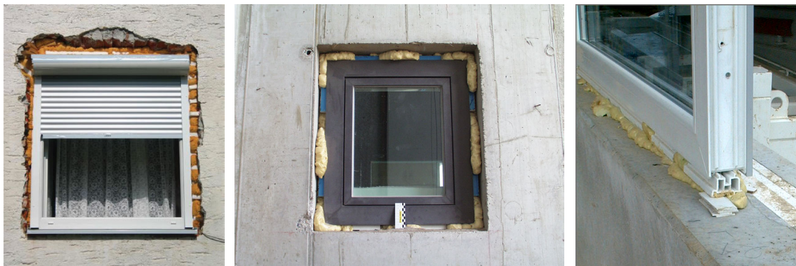
Figure 2 – Examples for bad window-wall connections
