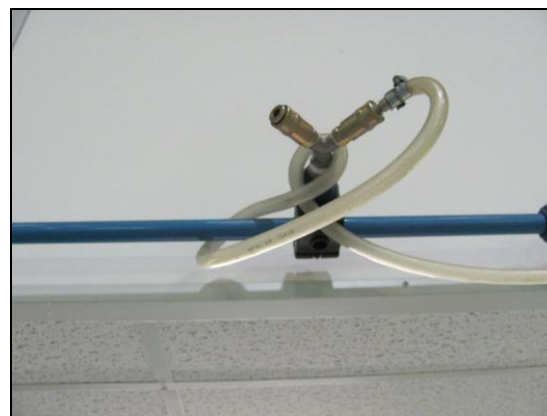
Figure 10. Leaky air attachment point
