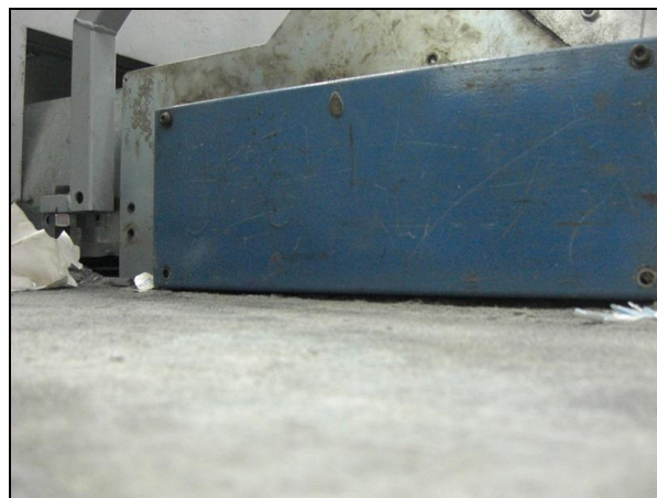
Figure 12. Waste chute panel missing two fixing bolts
