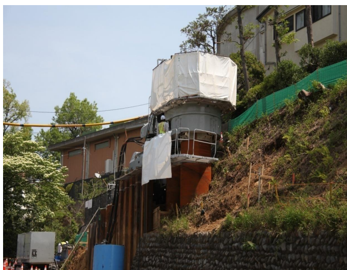
Figure 16 – Gyropress Hard-ground Press-in Method in Operation (Japan)
