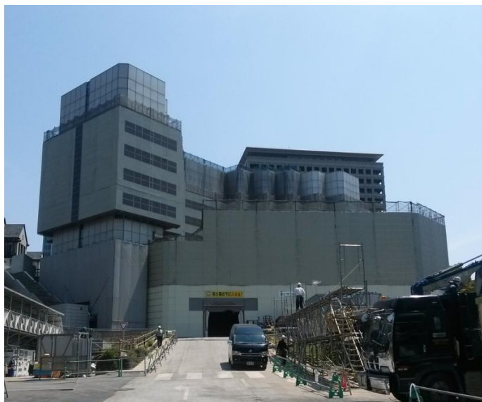
Figure 15 – Hat-down Demolition of Grand Prince Hotel Akasaka (Japan)
