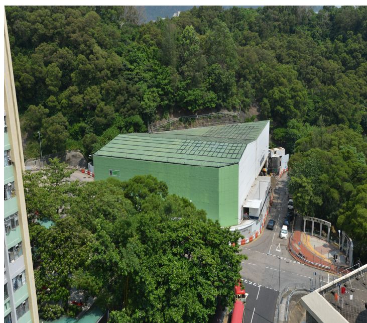
Figure 11 – Purposely-built Substantial Acoustic Enclosure
