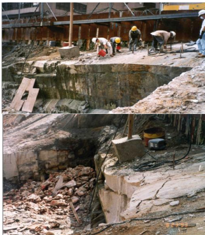
Figure 6 – Employment of Expandable Chemical Agents and Resultant Cracked Rocks
