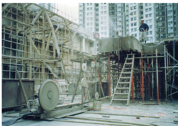
Figure 5 – Wire Sawing of Concrete Floor Slab
