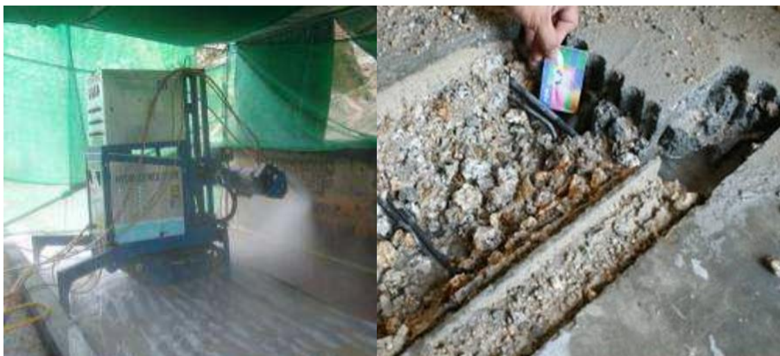
Figure 9 – Removing Concrete by Hydro-scarification (Source: Housing Department, HKSAR Government)
