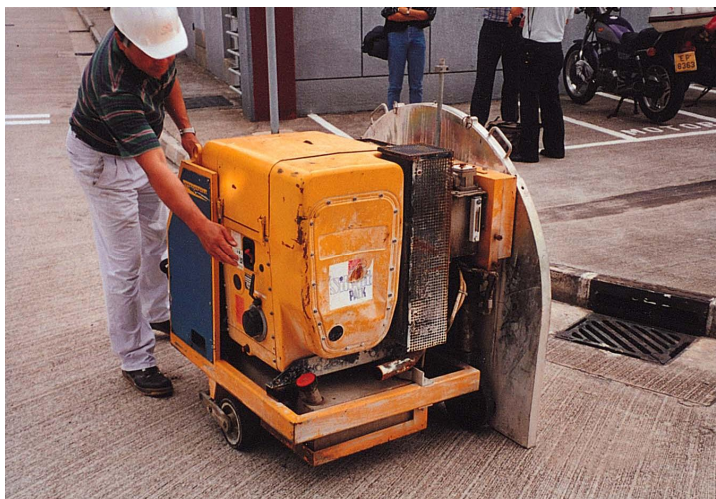
Figure 3 – Blade Sawing of Concrete Slab
