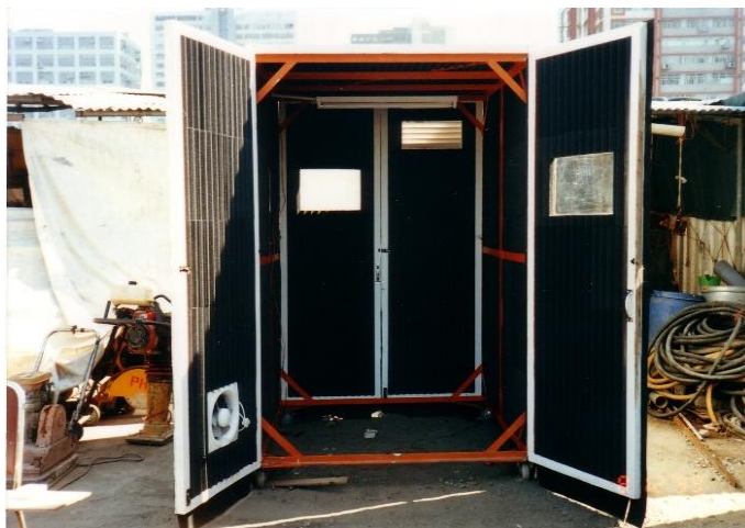
Figure 12 – Movable Enclosure with Internal Sound Absorption Lining
