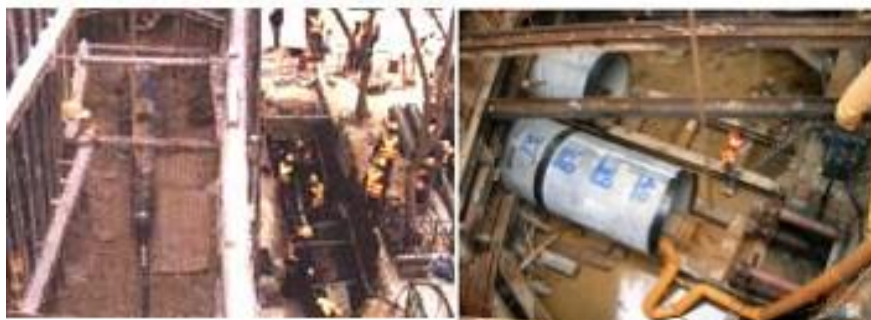
Figure 8 – Pipe jacking method (Source: Water Supplies Department, HKSAR Government)
