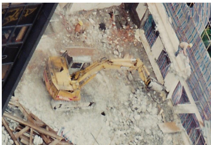
Figure 1 – Conventional excavator-mounted percussive breaker
