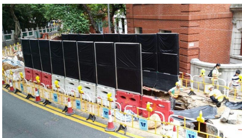
Figure 13 – Movable Noise Barrier
