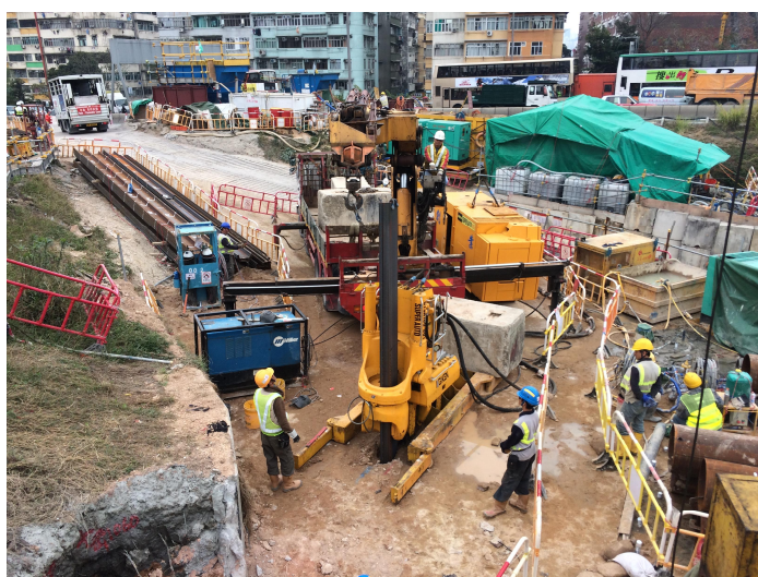
Figure 7 - Hydraulic Press-in Method
