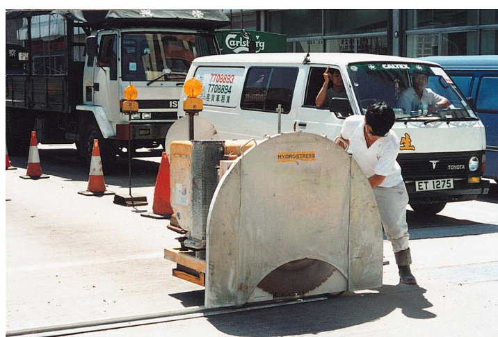
Figure 4 – Hydro Blade Sawing of Concrete Slab
