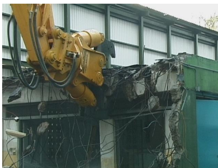
Figure 2 – Hydraulic crushers for demolition works
