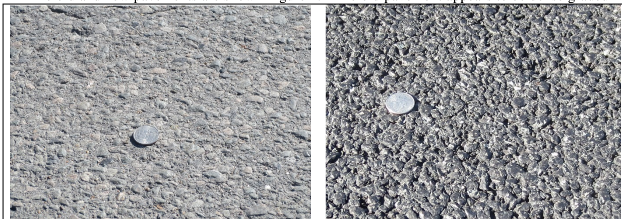
Figure 4 - Photograph of old dense grade asphalt (left) and new open-graded asphalt (right)
