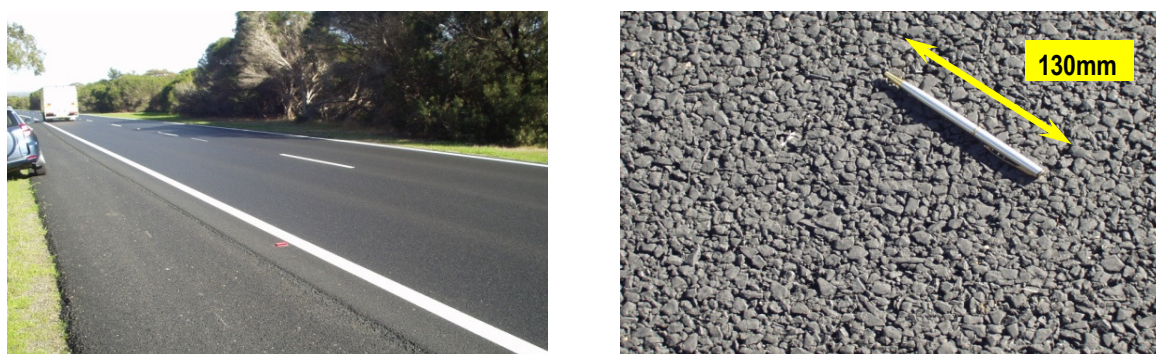
Figure 3 –Section 3 double layer OGA. (L.H.S.: the upper layer extends partly onto the emergency)
