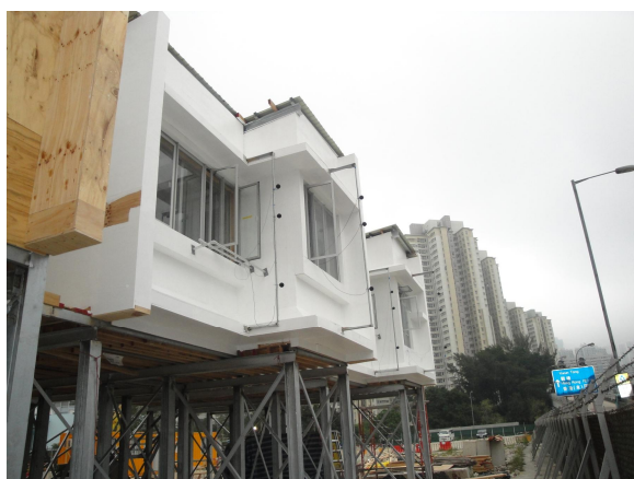
Fig. 4 - The mock-up flats for in-situ tests windows
