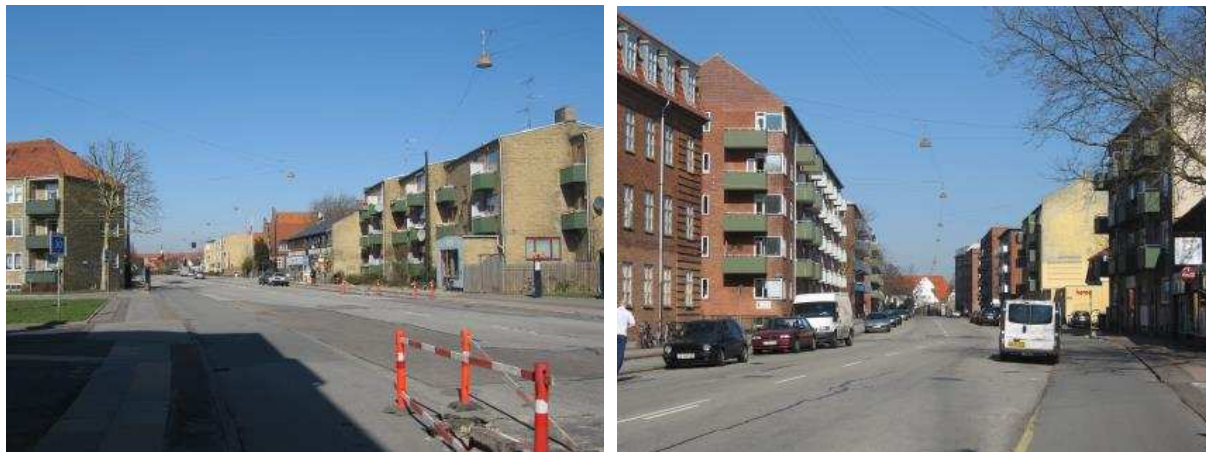
Figure 3 - Photographs from Kastrupvej before the replacement of the pavement.
