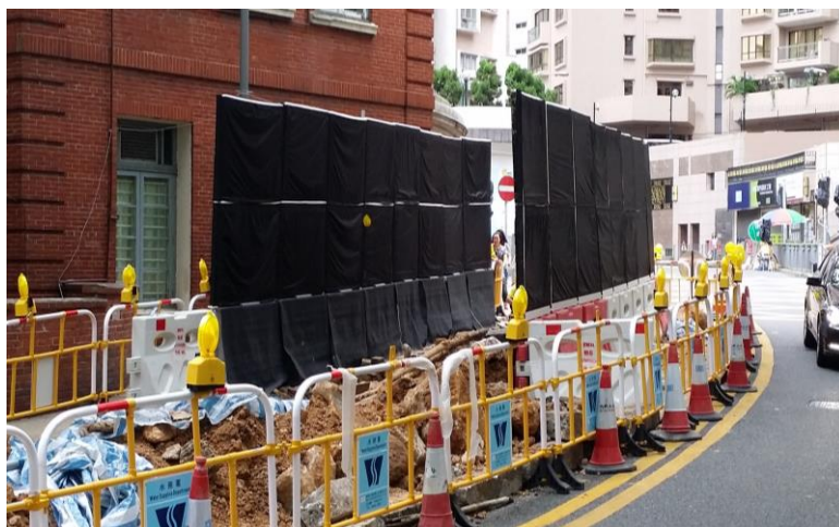
Figure 6.2 – Installation of barrier on one lane of the road.
