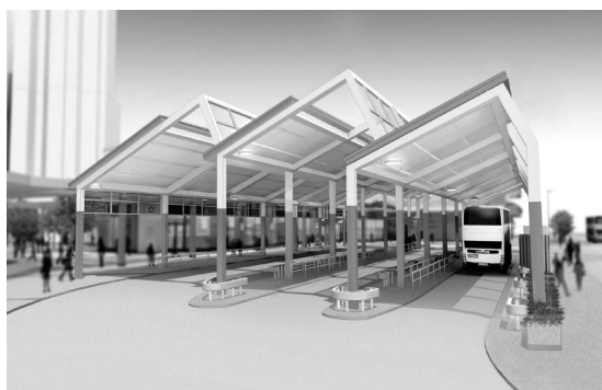
Figure 2: Noise Cover for PTI at Hung Shui Kiu Area 13
