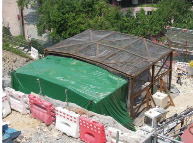
Figure 5 - Nissen Hut (with Blast cages inside)
