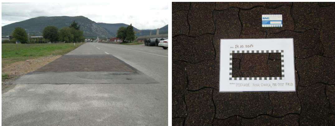
Figure 4 – The Slovenian pilot test track in Nova Gorica; prefab PERS on concrete setts (pictures: D. Kokot, ZAG)
