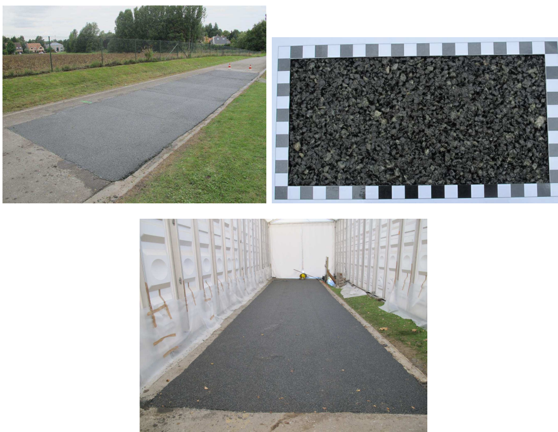
Figure 5 – The Belgian pilot test track in Sterrebeek; on site construction: Sterrebeek I (two top pictures) and Sterrebeek II, which had to be constructed under a tent due to the cold and wet season (lower picture) (size of black/white squares is 10 mm) (pictures: A. Bergiers, BRRC)
