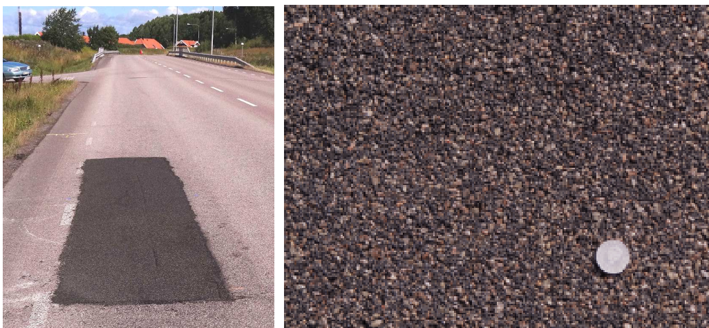
Figure 3 – The Swedish pilot test track in Linköping; on-site construction (pictures: U. Sandberg, VTI)
