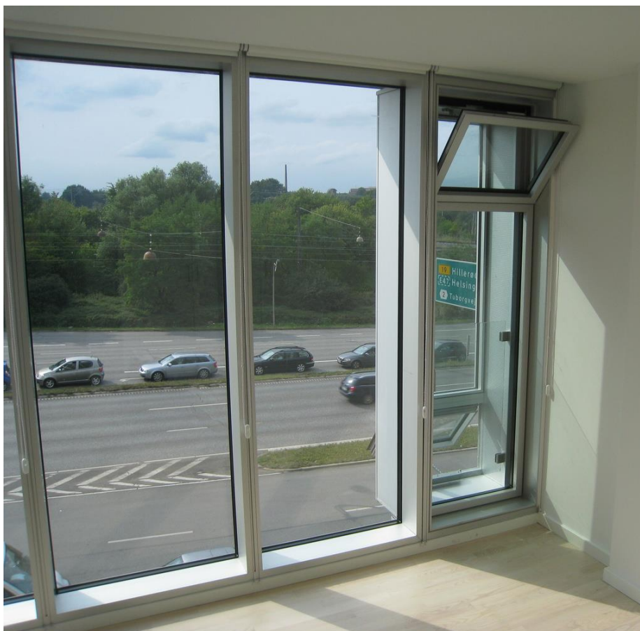
Figure 3 – View towards the noisy road with (from the left) two non openable window sections and one Supply Air Window with open vents
