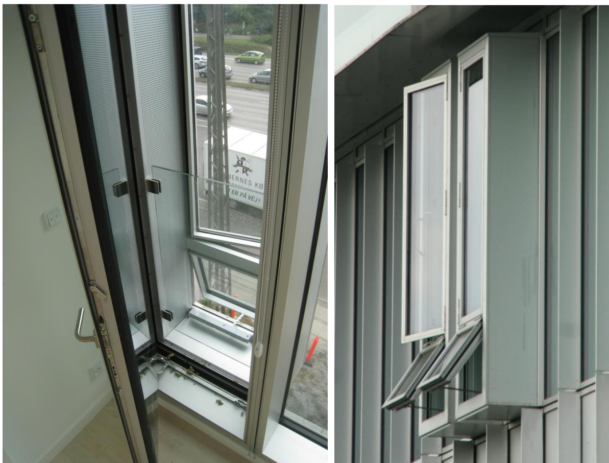
Figure 4 – Left figure: View out through the Supply Air Window with both service openings open and vents open. A security glass panel is also visible. Right figure: Two Supply Air Windows seen from the outside next to each other. For both windows the bottom vent is open, where it is only the left Supply Air Window who has an open service opening.
