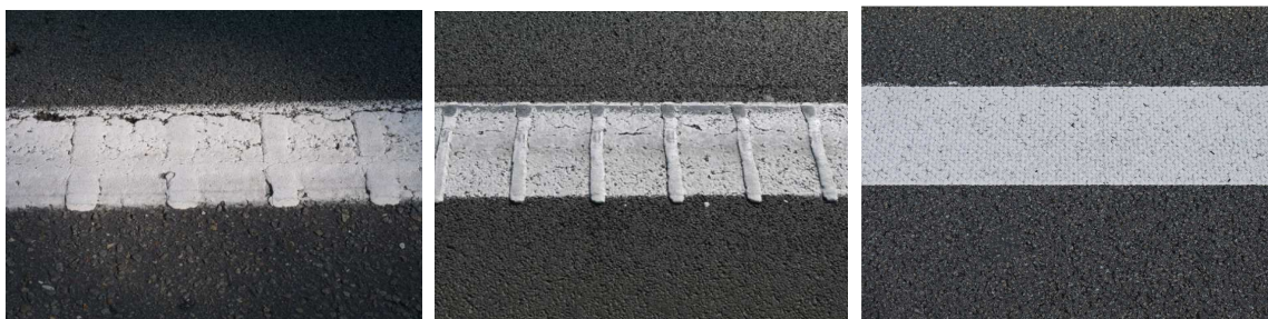
Figure 4 – Some tested audio-tactile road markings with dots (upper row) and ribs (lower row, left and middle) and tape with diamond pattern (lower row, right hand side)
