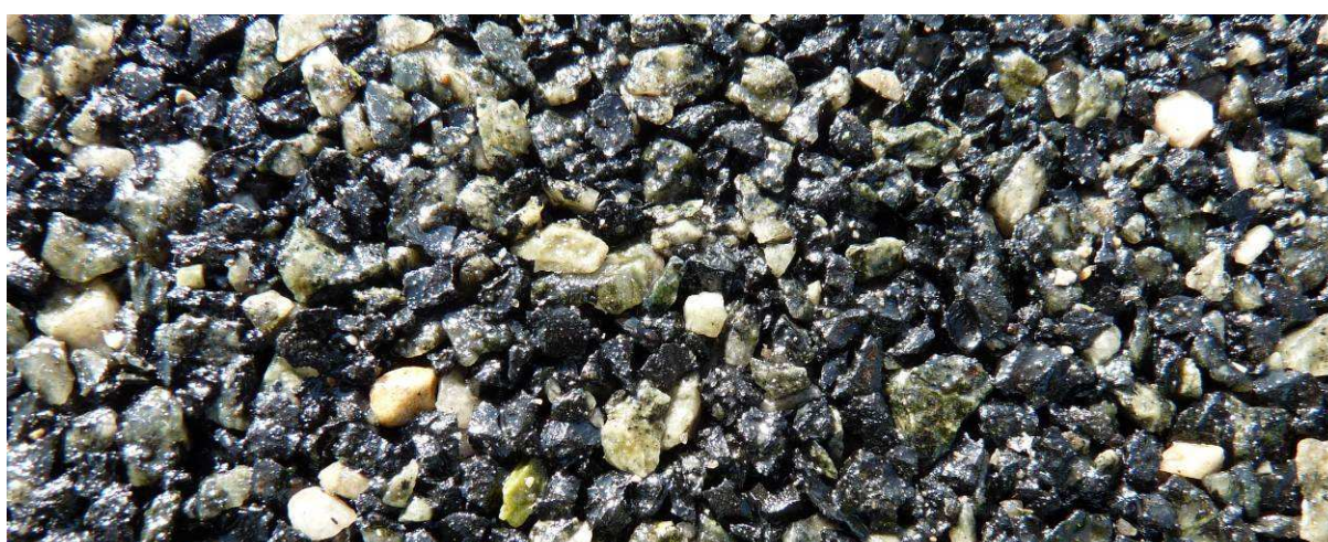
Figure 2 - Close up photo of the PERS test section. The light aggregates are stone material and the black are rubber material.
