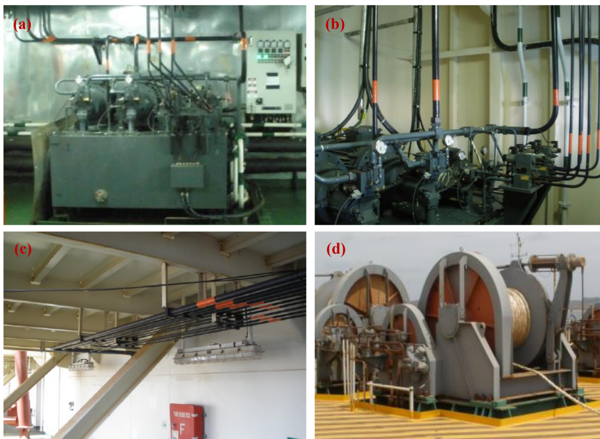
Figure 1 – Marine hydraulic mooring winch system comprised of (a) hydraulic power pack (HPP) unit, (b) & (c) hydraulic flow pipes and (d) mooring winch units.
